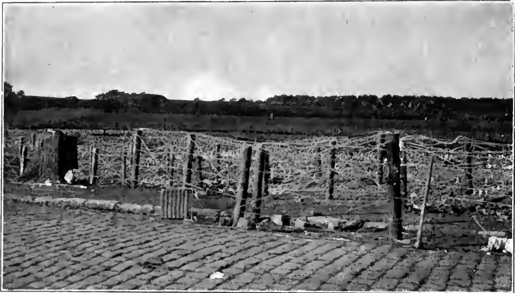
ELECTRIFIED BARBED WIRE ENTANGLEMENT OUTSIDE THE CITY.
